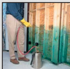
Treat the sill, band joists, subfloor and floor joists in a crawl space or basement structure.
