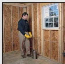
Treat the inside of an exterior wall and sheathing.
