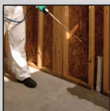
Use optional marker dyes for quality control and to ensure proper application.
